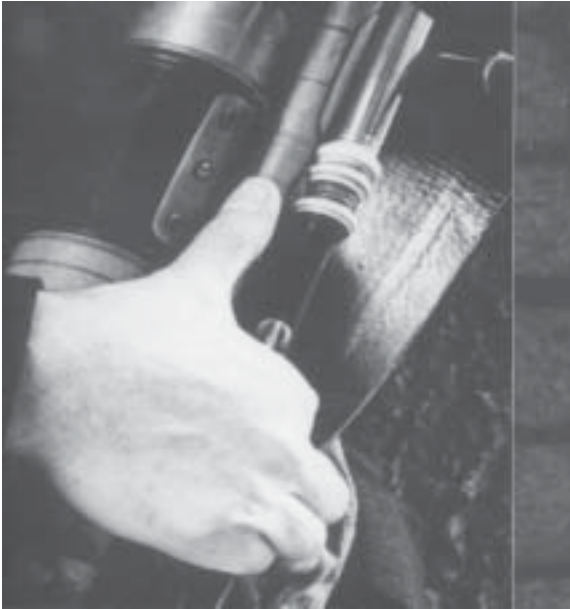
4-345 Pipeline - Dermot Hyde & Tom Hake
